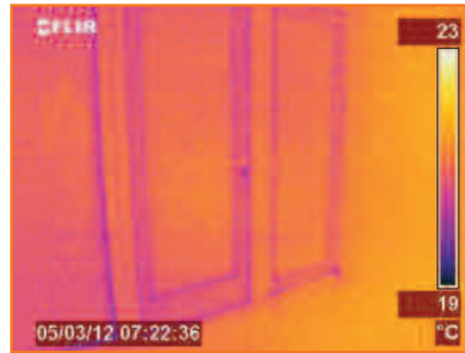
Above: A thermographic picture of the inside of the windows on a cold day; the temperature on the glass is high meaning it is comfortable to sit next to.
